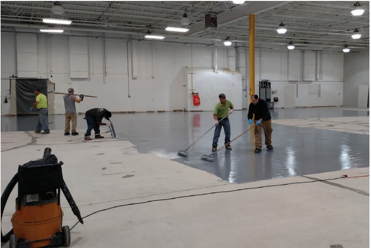
Fig 5. Crew applying EPOX-Z IC with squeegee and rollers
