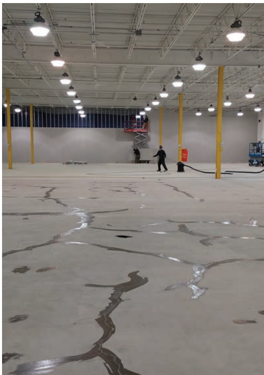
Fig 3 & 4. Repaired cracks with EPOX-Z Mastic
