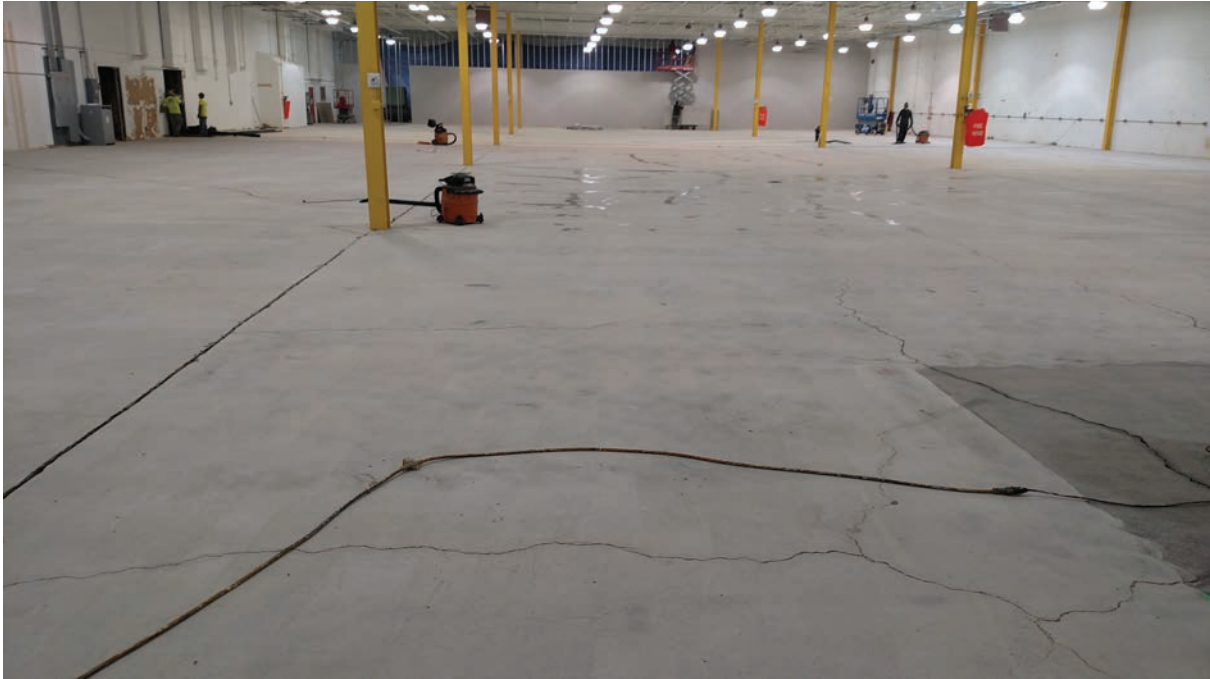
Fig 1. 27,000 sq. ft. floor has been cleaned and prepared for coating
