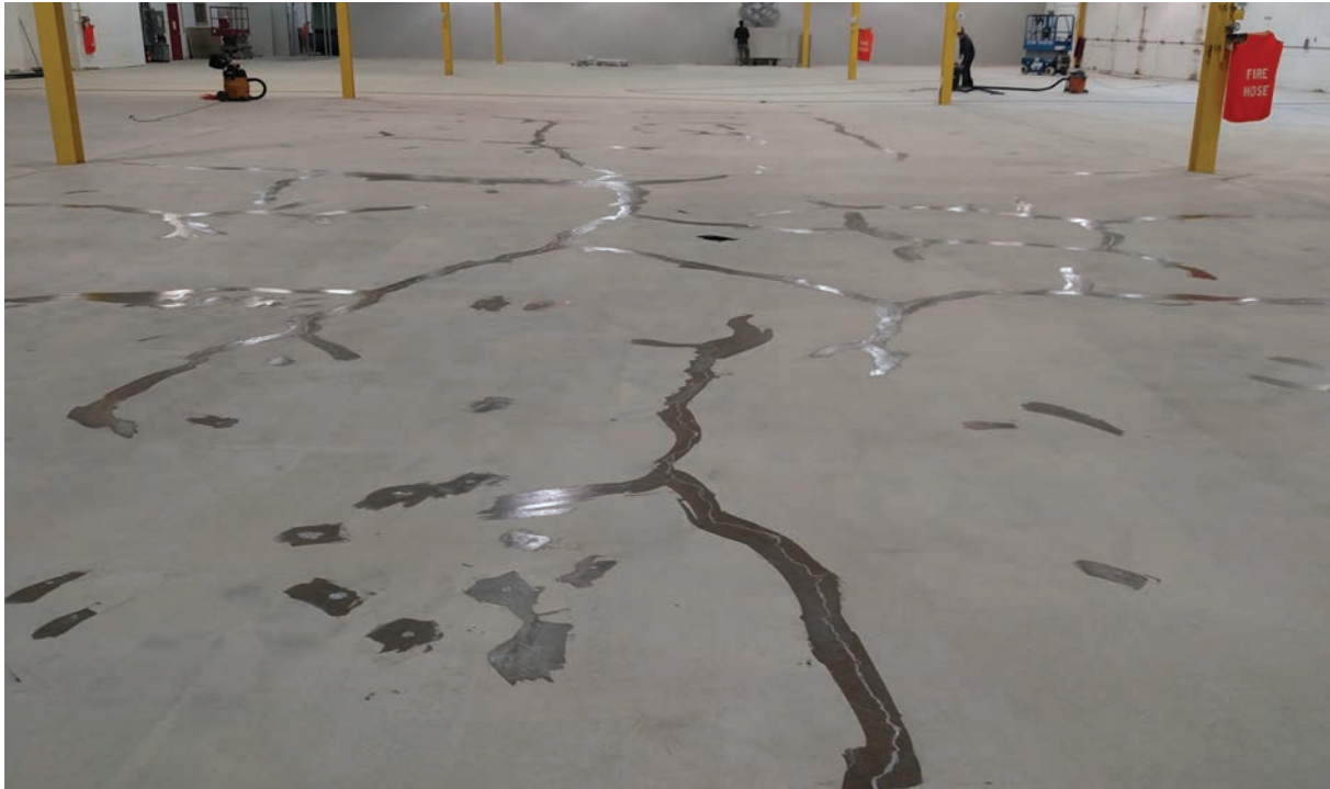
Fig 3 & 4. Repaired cracks with EPOX-Z Mastic
