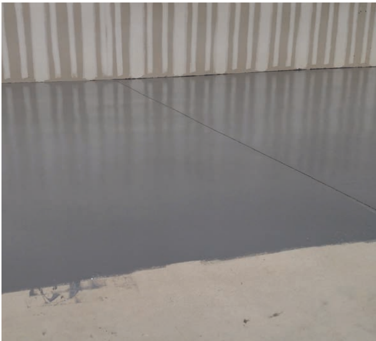
Fig 6. Completed section of floor
