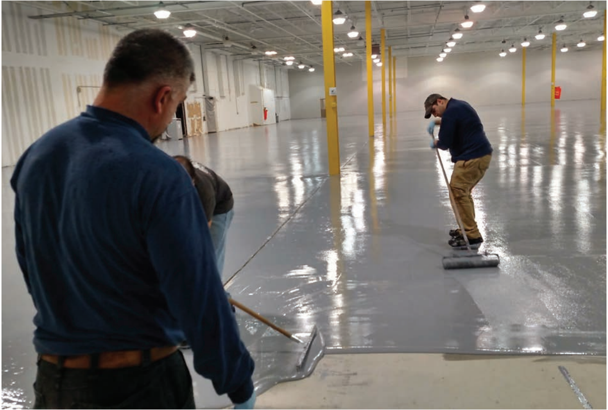
Fig 7. Application being completed
