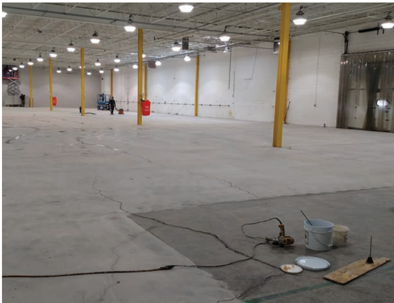
Fig 2. Crack repair with EPOX-Z Mastic begins
