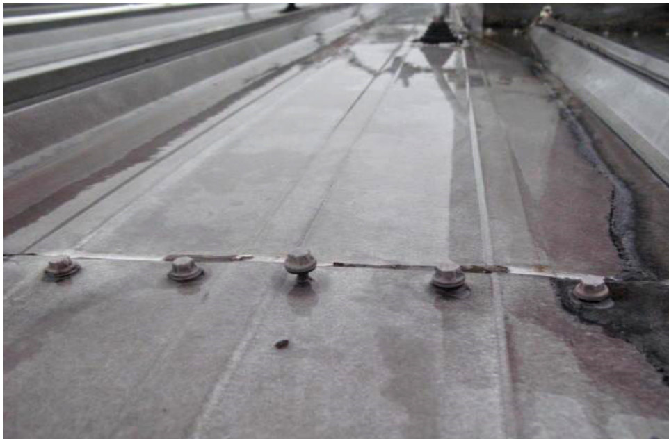
Fastener Back Out
